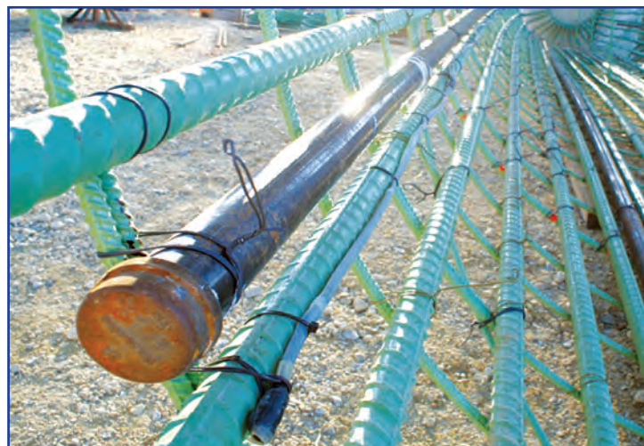
Thermal Wire™ attached to rebar cage (shown adjacent to access tubes.)
